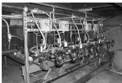
These high and intermediate pressure automated RSVP-UC valves have been in successful operation for 8 years. Installed at a cogeneration gas fired plant on the east coast, these valves have fail-safe actuators with jack-screw override.
